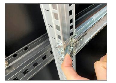
Position the slide rail assembly in your rack and align the mounting bracket to the rack posts. Then pull the metal clip and place the slide rail assembly onto the rack posts.
